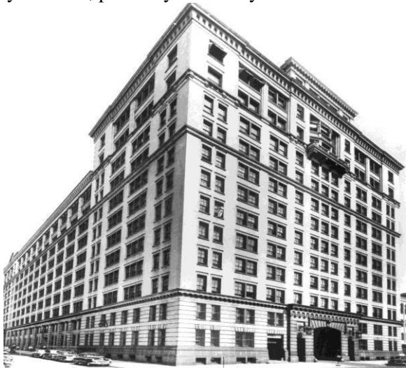
Figure 1: The original home of Bell Laboratories beginning in 1925, 463 West Street, New York.
